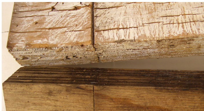
Azotek treated (Bottom) and untreated samples from framing trial.
